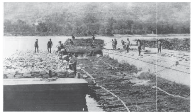
Throwing Rock on Brush Mats. Photograph by Henry Bosse, 1891 Source: U.S. Army Corps of Engineers
