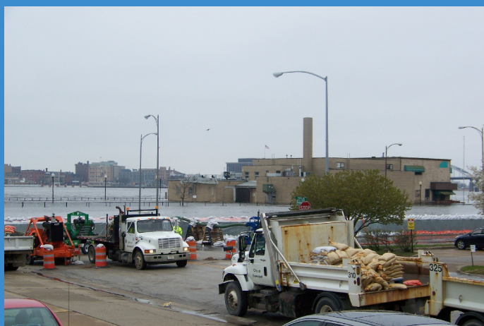
Flood Fighting in Davenport, Iowa, in 2007. Photo by Brad Walker.
