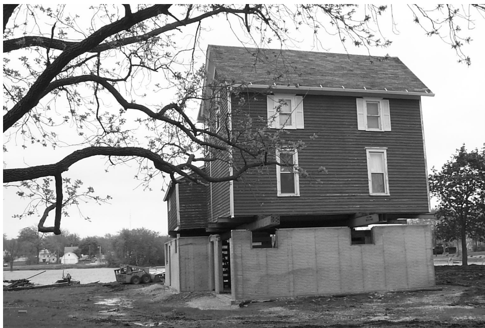
At first, said Joni Hocken, their Independence, Iowa, neighbors were puzzled by the spectacle of their 100-year-old, two-story, red-painted home being elevated on new concrete foundation walls. (Photo: Mike McCoy, FEMA)
