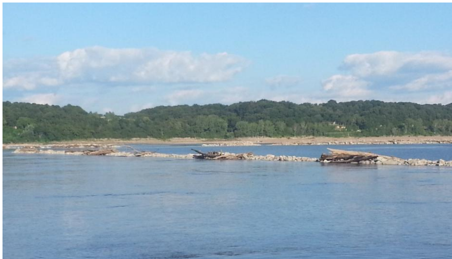
Figure 1: Wing Dikes constructed along the Missouri River during the BSNP
